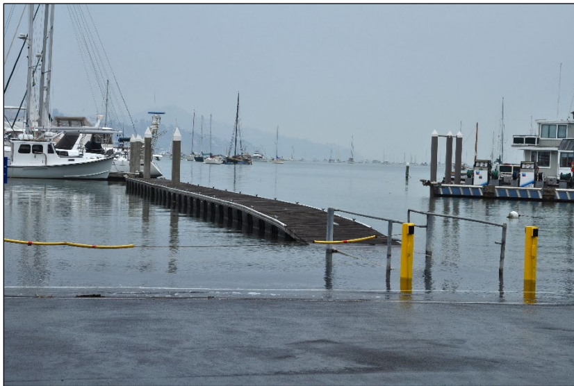
Figure 10: Example king tide flooding impacting access to float, CCC (2019).
