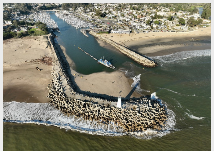
Pictured above, Twin Lakes working extended hours to address entrance channel shoaling on January 20, 2023.
