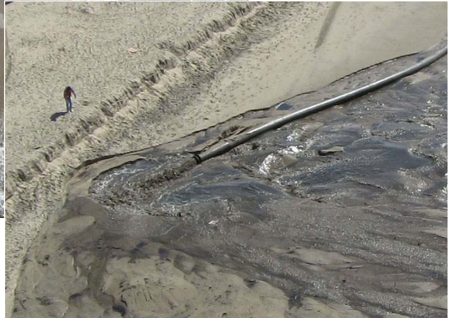
Figure 7. Sand Placement on Beach
