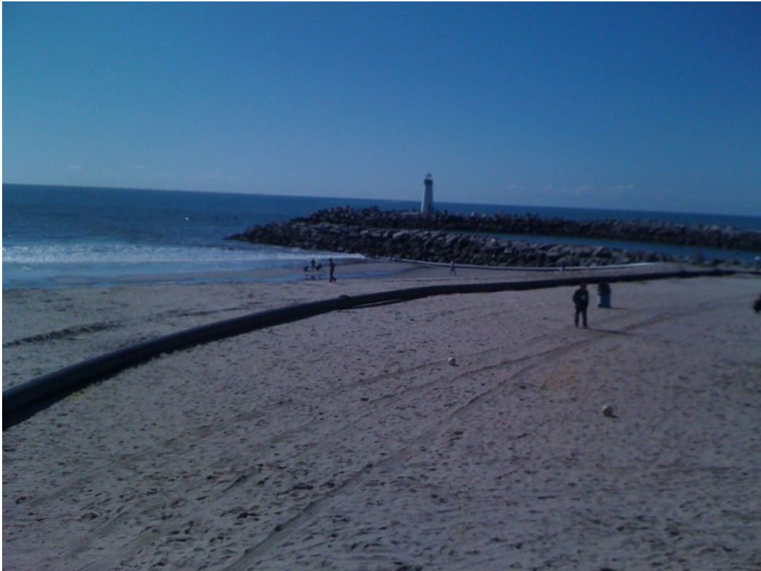
4. Beach Replenishment Underway
