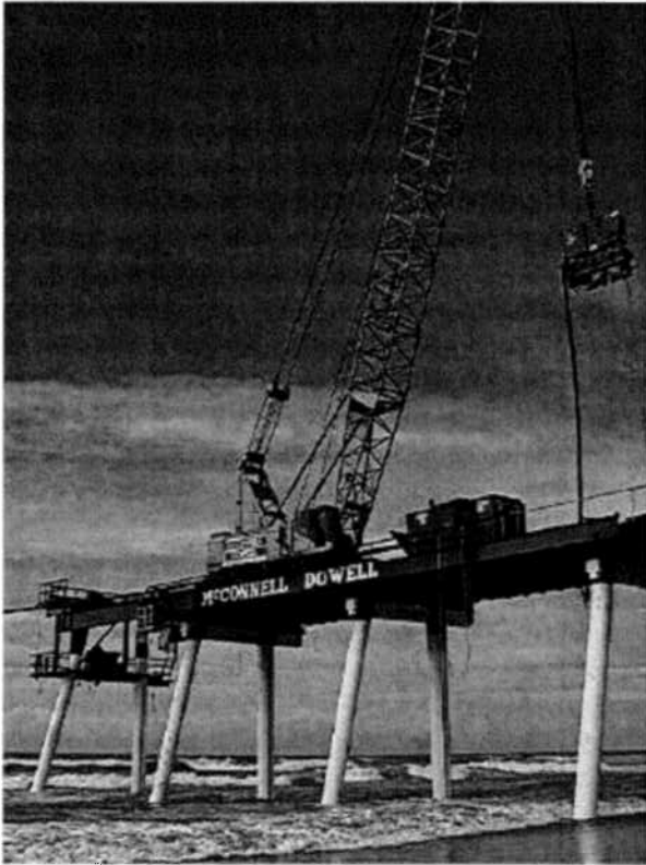
Jetty under construction
