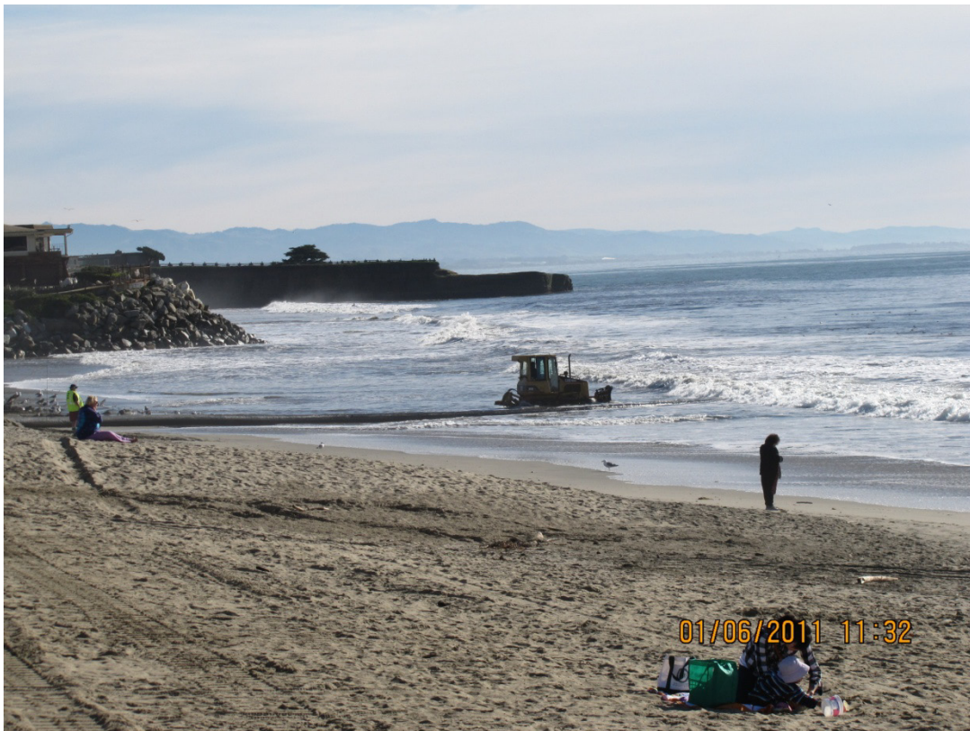
2. Beach Replenishment Including Tractor Operations Underway
