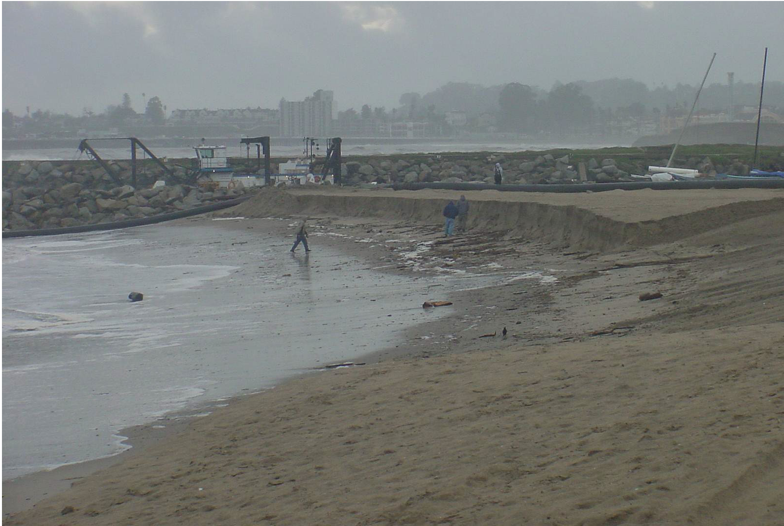
Figure 3. Erosion of Newly Placed Sand at Beach East of Jetty, March 24, 2011.
