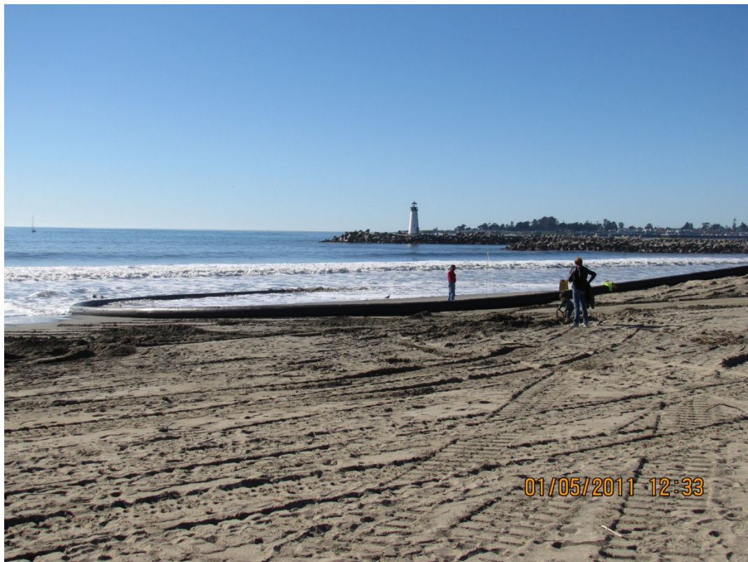
1. Beach Replenishment Underway
