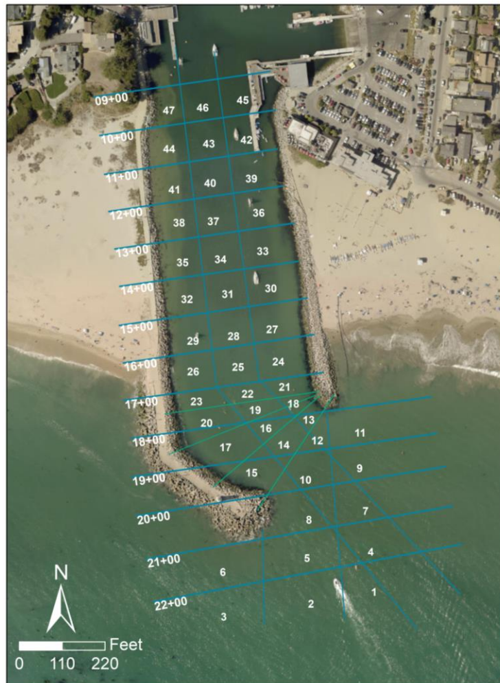
Figure 8 Dredging Quadrants for Harbor Entrance (recreated from Santa Cruz Harbor District, 2014)
